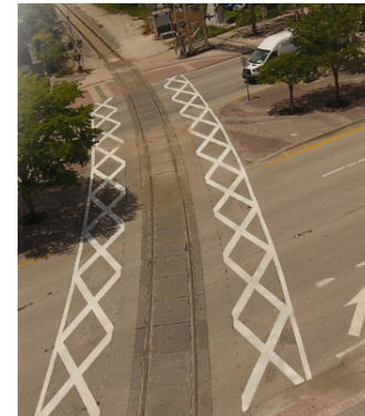
Figure (left): Sample DO NOT STOP ON TRACKS signage Figure (right): Sample dynamic envelope pavement markings
