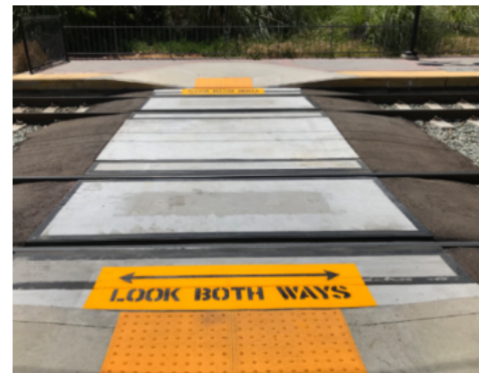
Figure: Example of tactile warning and pavement marking
