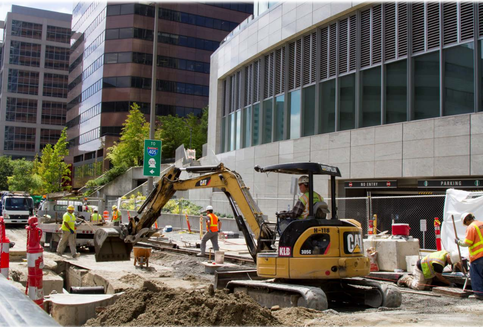
Downtown Bellevue north portal construction
