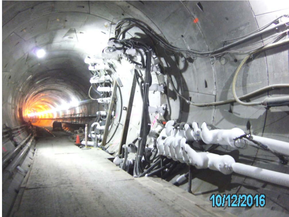
Soil freezing technology to stabilize soil
