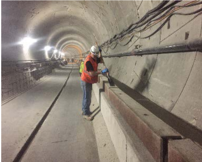
Walkways, fire standpipes, lighting & conduits
