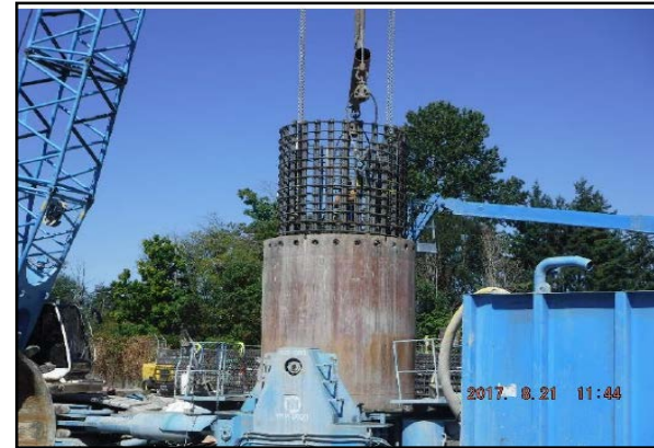
Drilled Shaft in Bel-Red
