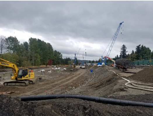
Site preparation for Station and Garage
