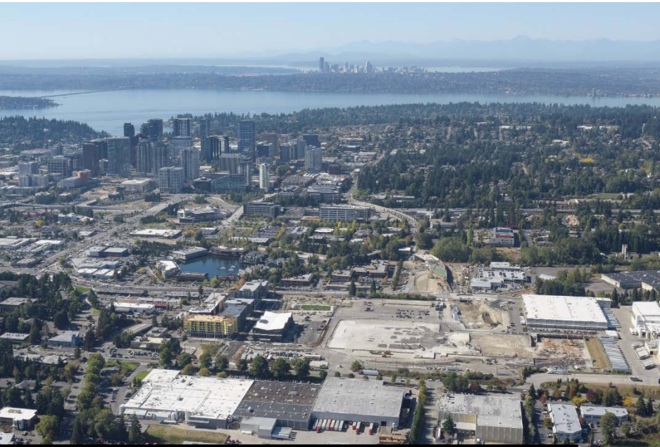
Aerial provided by Wright Runstad – looking west
