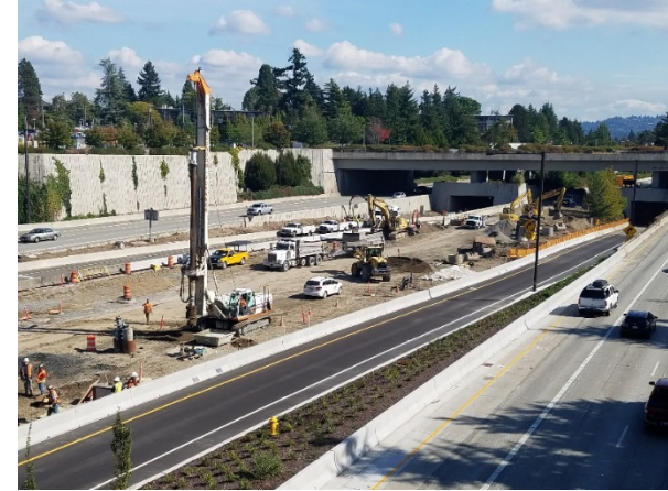
Site Work and Foundation Construction at Mercer Island Station
