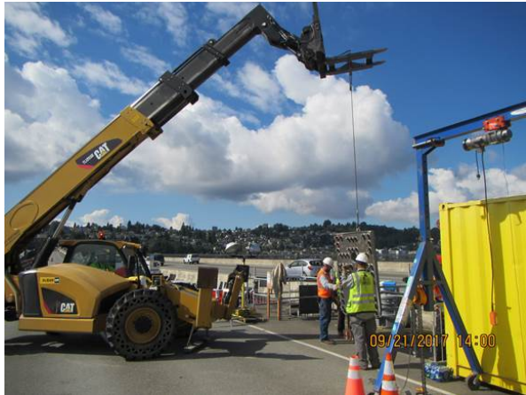
Anchor Frame Placement in I-90 Bridge Pontoon
