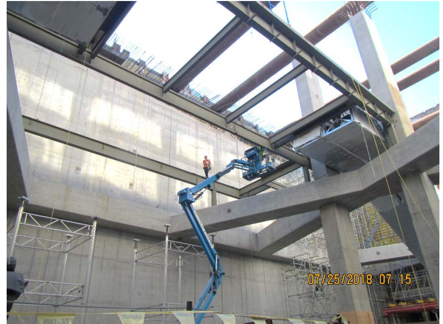
Mezzanine Steel Installation
