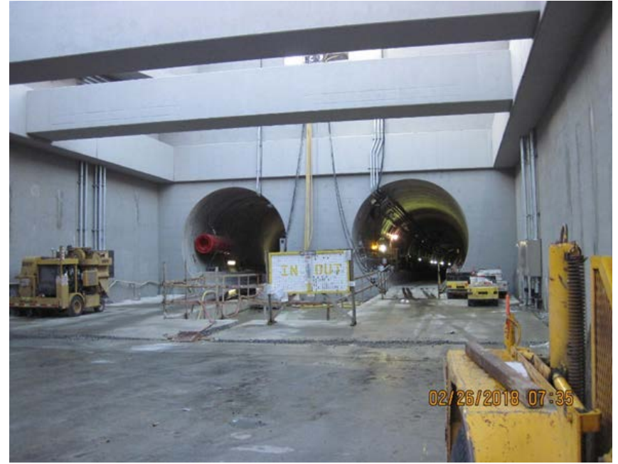
Completed Maple Leaf Portal
