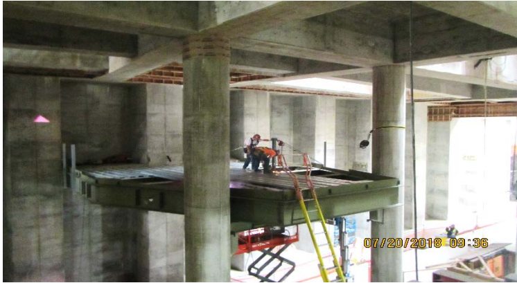
Mezzanine stair platform installation
