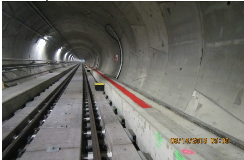
Rail installed under UW Campus
