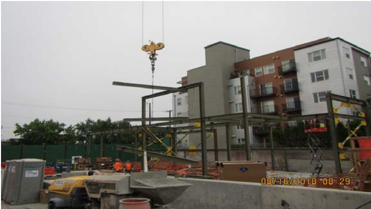
South entry steel installation
