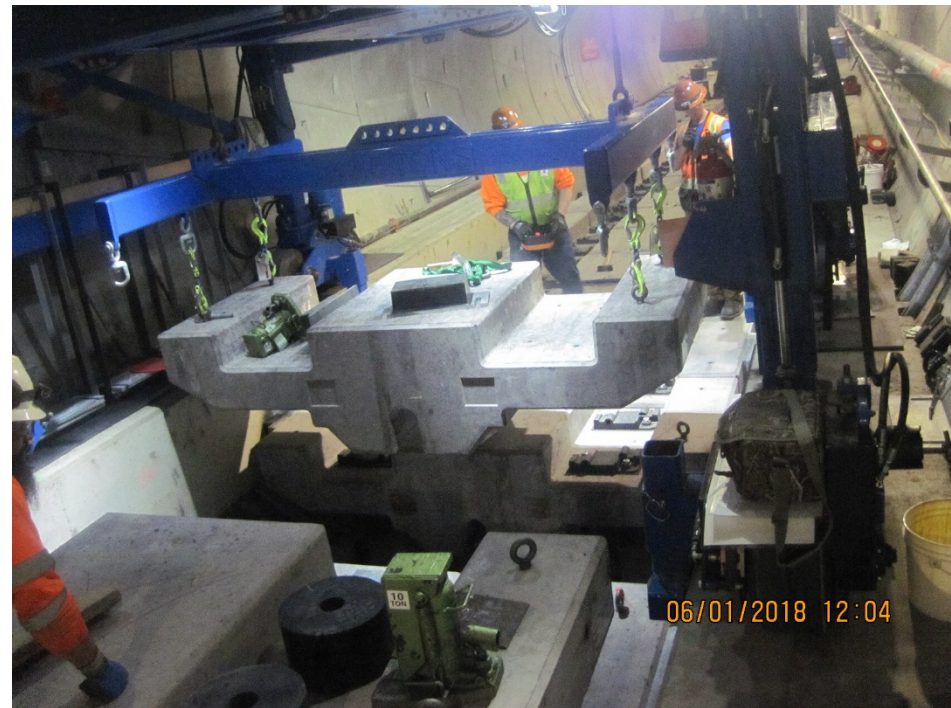
Installing floating slab
