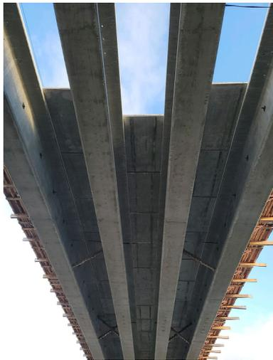
Guideway precast panels placed between girders
