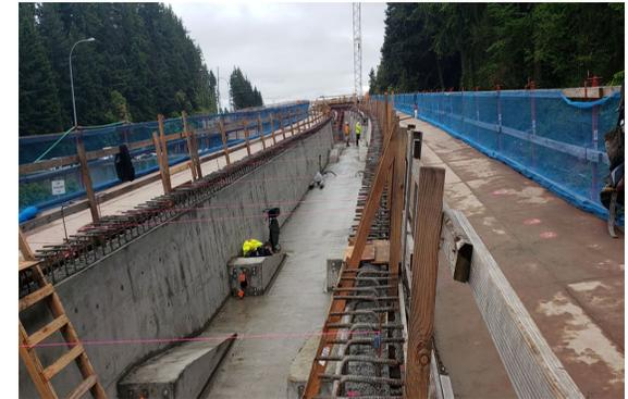
Cast-in-place tub girder concrete at I-5 overcrossing
