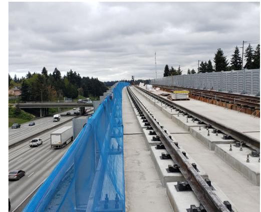
Elevated guideway direct fixation track installation in North Seattle
