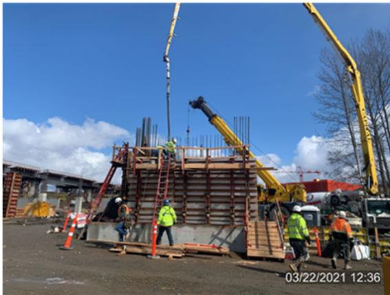
Placing shear wall concrete at the Lynnwood Station Garage
