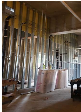
Interior framing and mechanical rough-in at the Mountlake Terrace Station ancillary buildings
