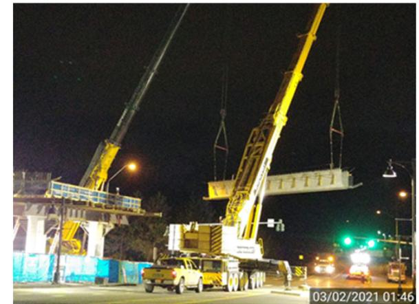
Girder installation over 236<sup>th</sup> St SW, east of I-5 at Mountlake Terrace Station
