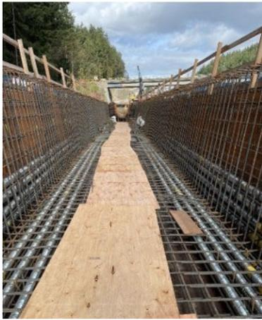
Rebar placed for I-5 overcrossing stem walls
