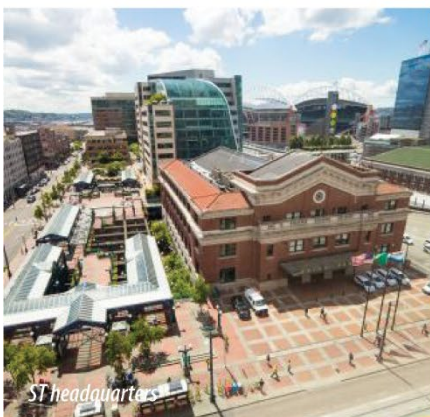
SCC 30 - Support Facilities
