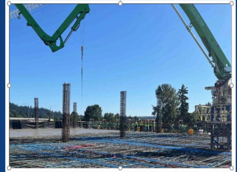
Downtown Redmond Link Extension Garage Construction
