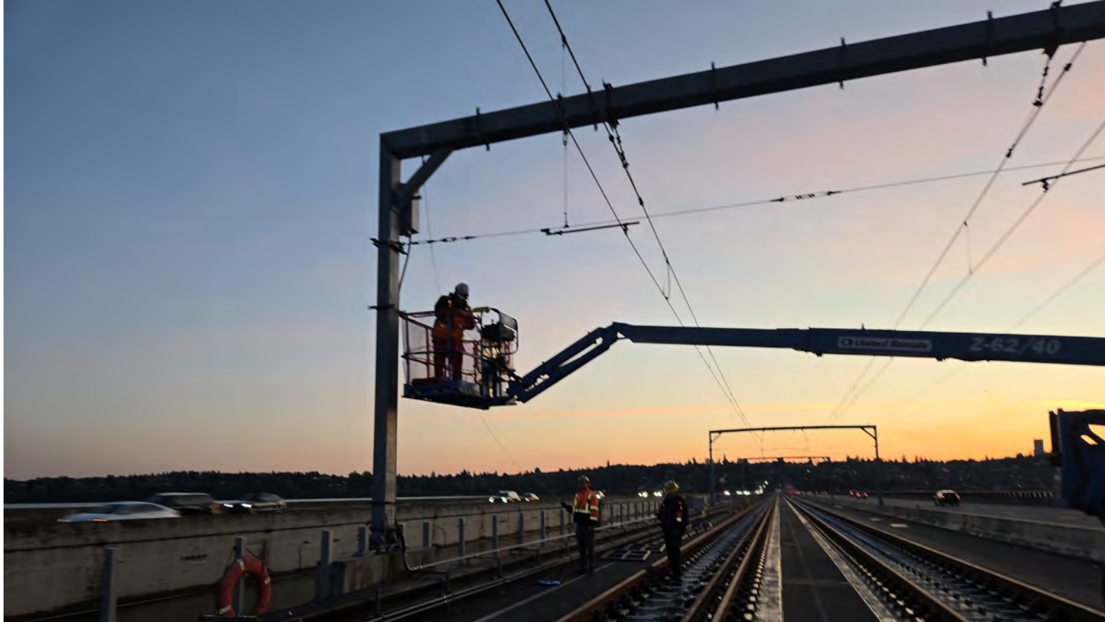
Overhead Cable Installation Along Floating Bridge (Systems)
