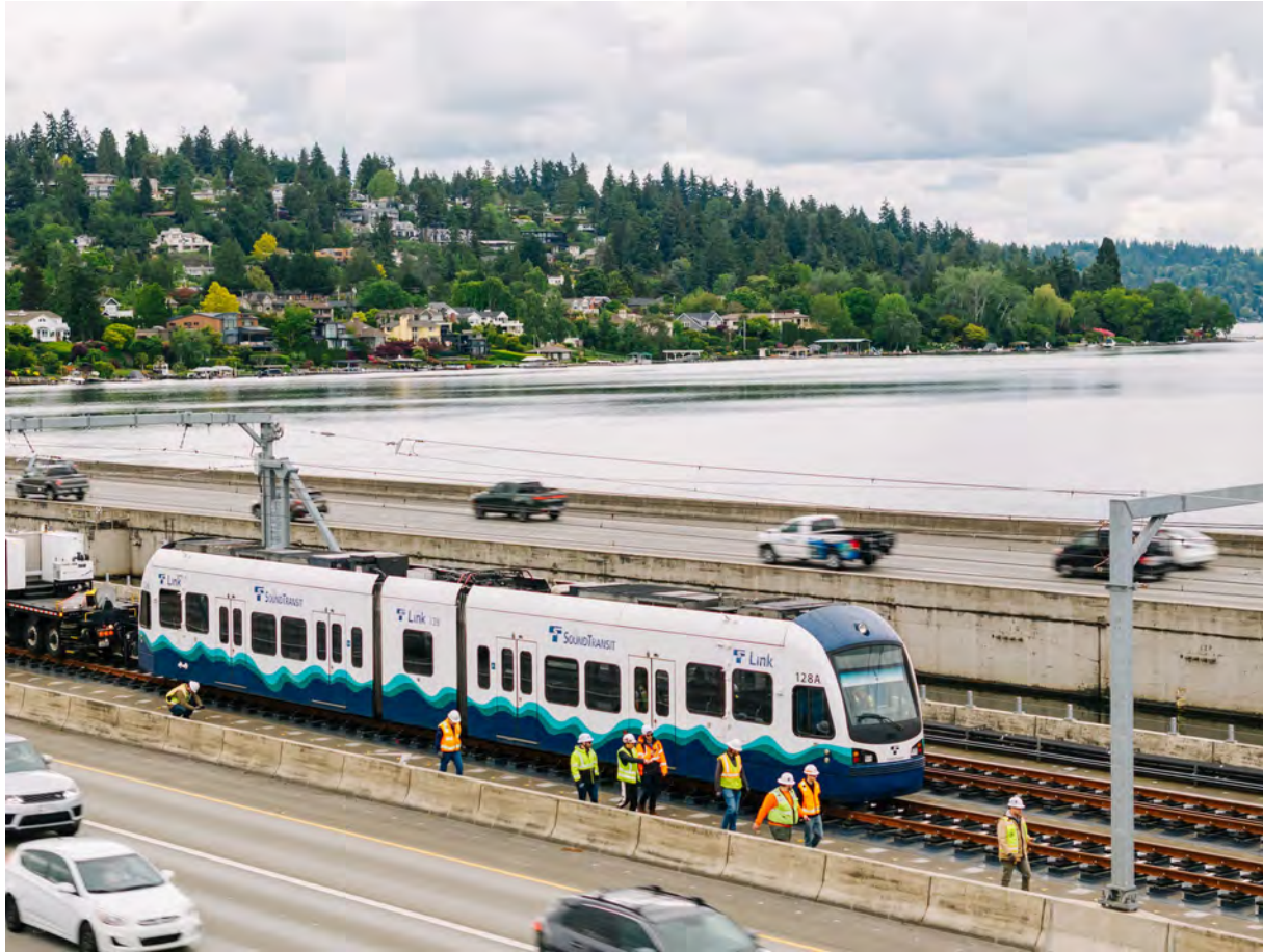
Floating Bridge Trackwork & Overhead Catenary
