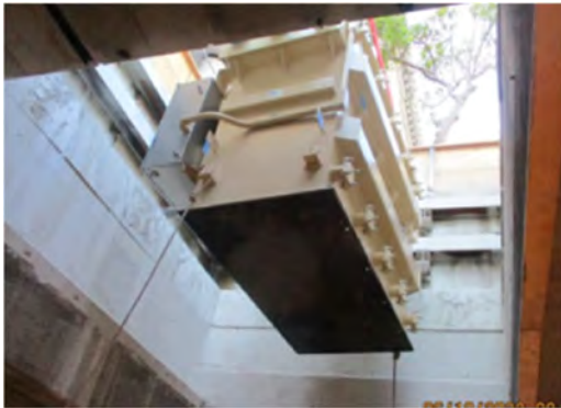
Figure 1 - New electrical infrastructure being installed through street access point in San Francisco.
