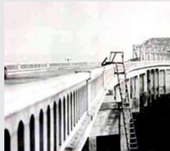
Puyallup Ave Bridge Construction (1926) Source: National Archives and Records Administration
