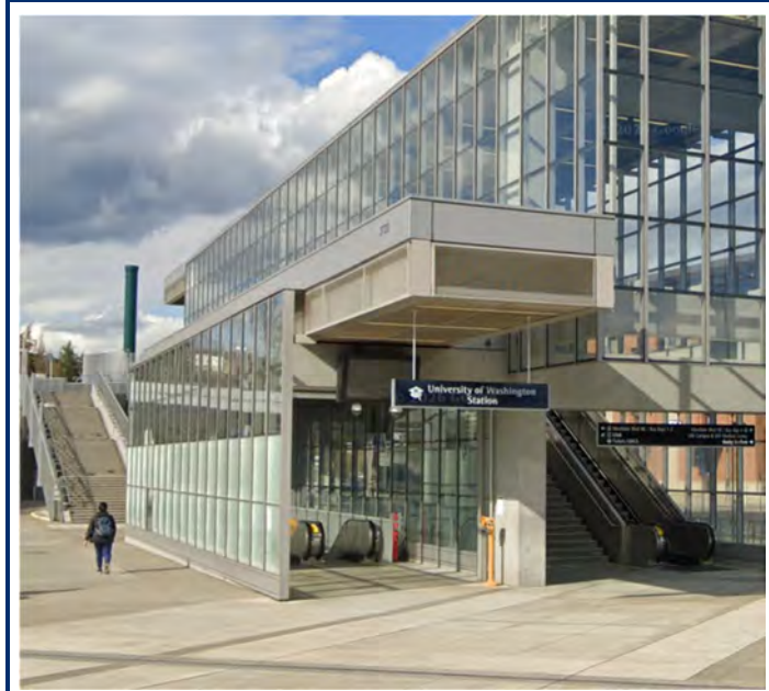
Figure 21-16 – University of Washington Station Existing Canopy to be Widened and Extended
