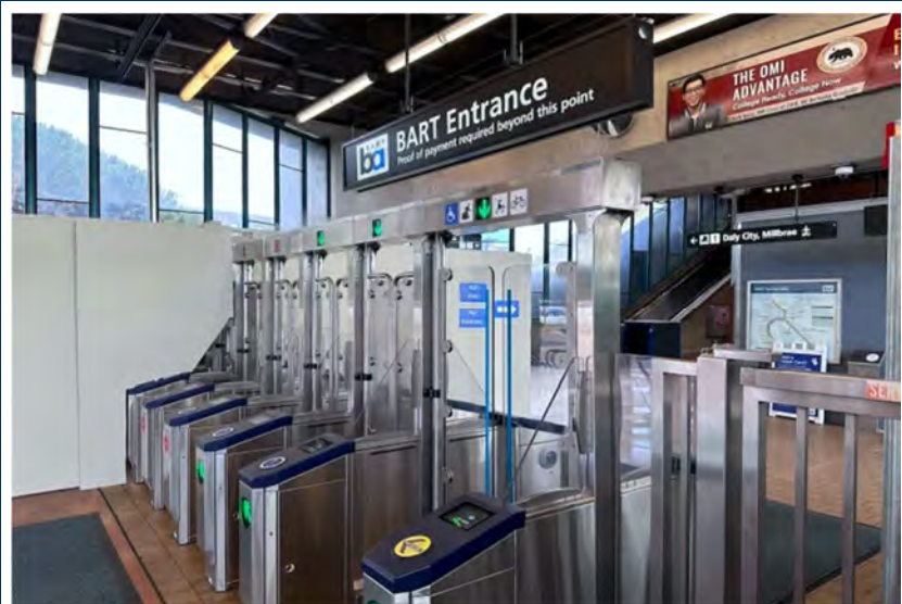
Figure 20-4 – Temporary Fencing at BART Gate Array
